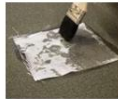
Joint Tape embedded into Primer
