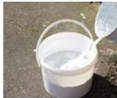
Catalysed product poured into aggregate
